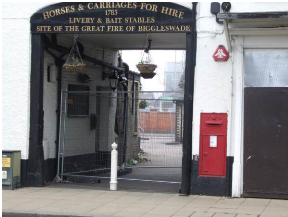
High Street - fencing across passageway
