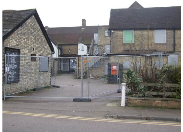
Church Street – fencing across car park entrance
